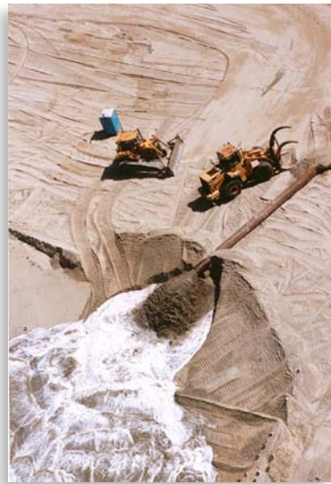
Bulldozers and sand at Batiqitos RBSP I
