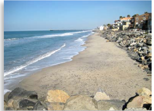
Oceanside at present
